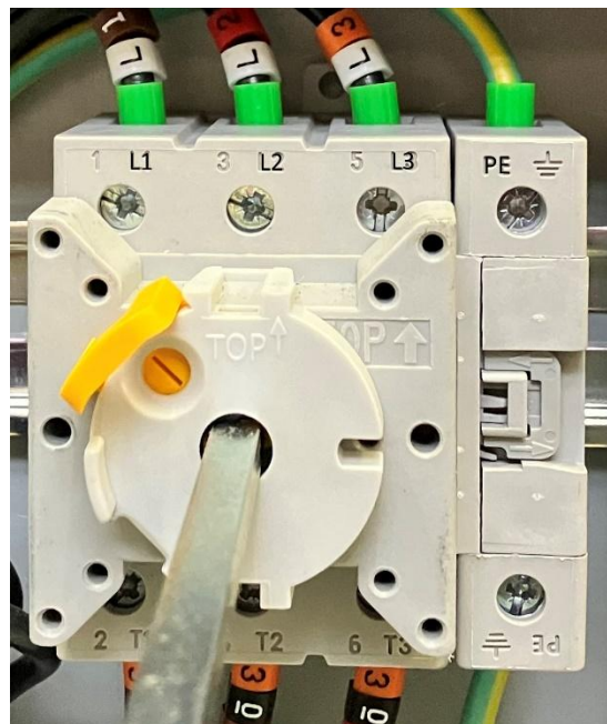
Figure 7 - Electrical connection of the machine
